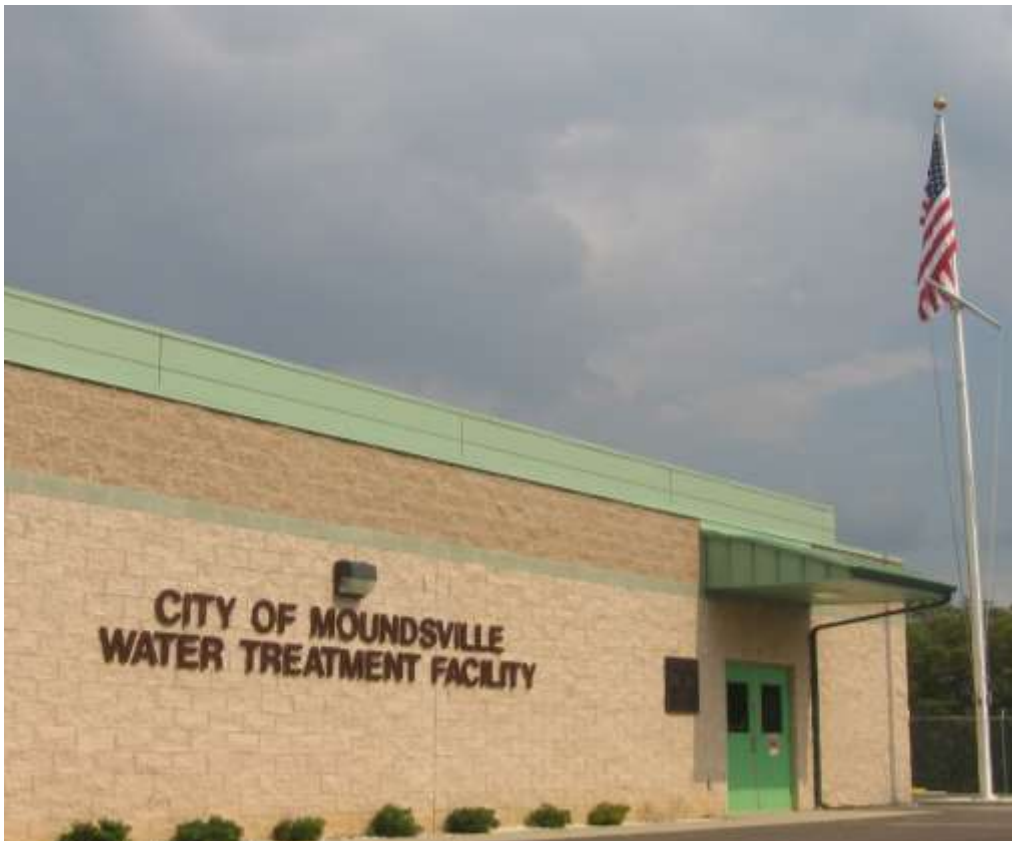
Water Treatment Plant - Front View Along Ohio River Completion Date: January 2008
